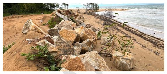
Figure 2-6 Eroded foreshore on northern tip of Cullen Point, with emergency seawall works partly buried by recent accretion
